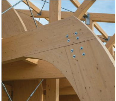
Bolted/ Doweled Connections
