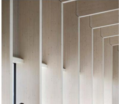
Glulam Timber Ribs
